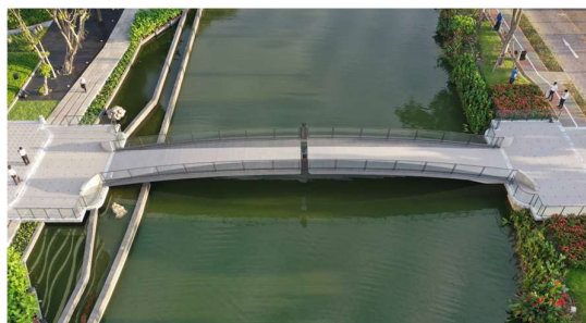
Fig.2. SCG-UHPC bridge at SCG Headquarter
