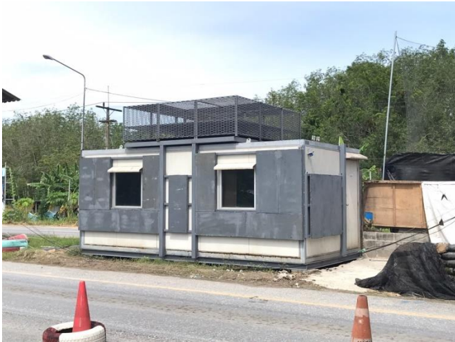
Fig.10. Buildings installed the bulletproof panels from the study.
