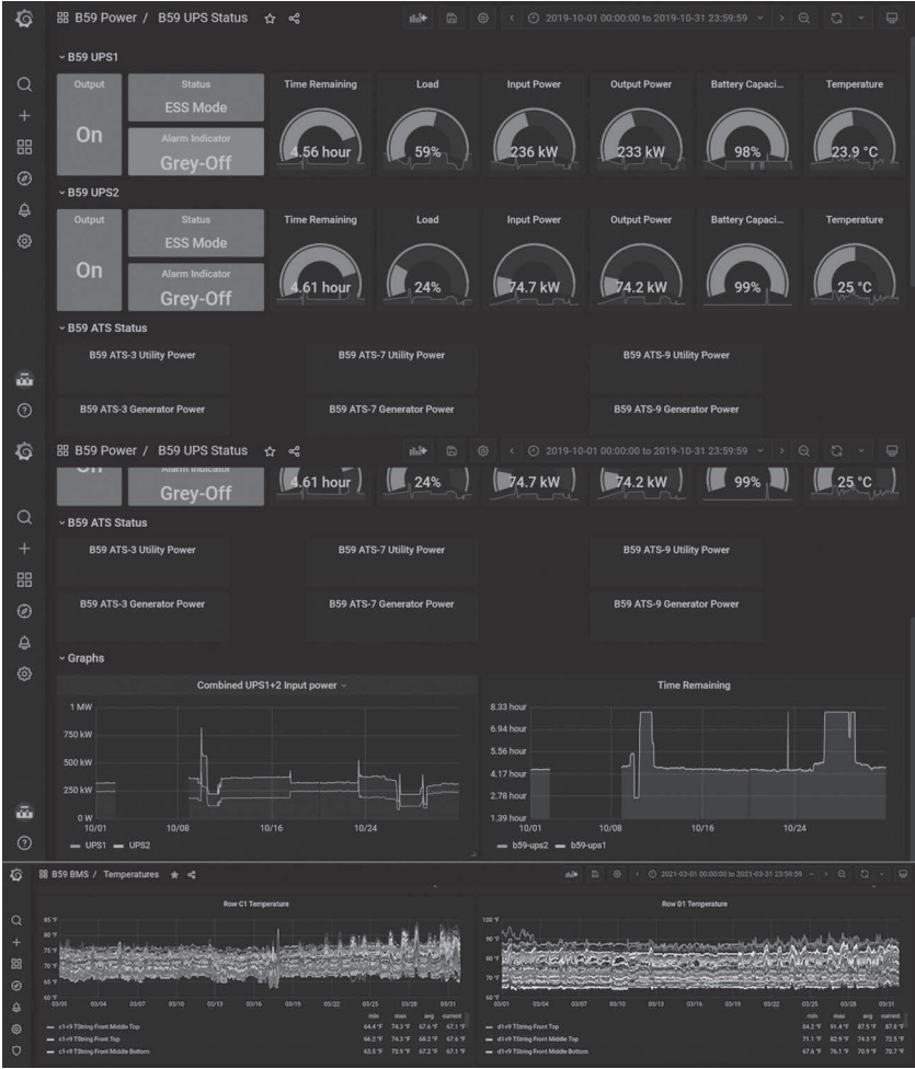
Figure 3.8 The three panels above show data points being monitored during PSPS. Panels 1 and 2 show the load on the UPS at that moment, and since the generator is not active, it has no load. Panel 3 shows the row and rack temperature fluctuations for Row C1 and Row D1.
