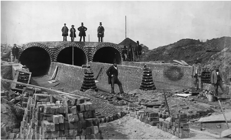
The Great Stink of 1858 – Main drainage of the metropolis. (Illustrated London News [London, England] 27 Aug. 1859 203.)
